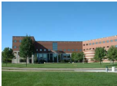
Pic. 2: Curris Business Building
